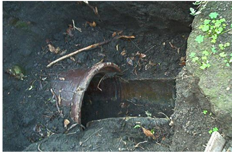
Ceramic culvert pipe discovered in a backyard on Milvia Street, along the Schoolhouse Creek channel.
