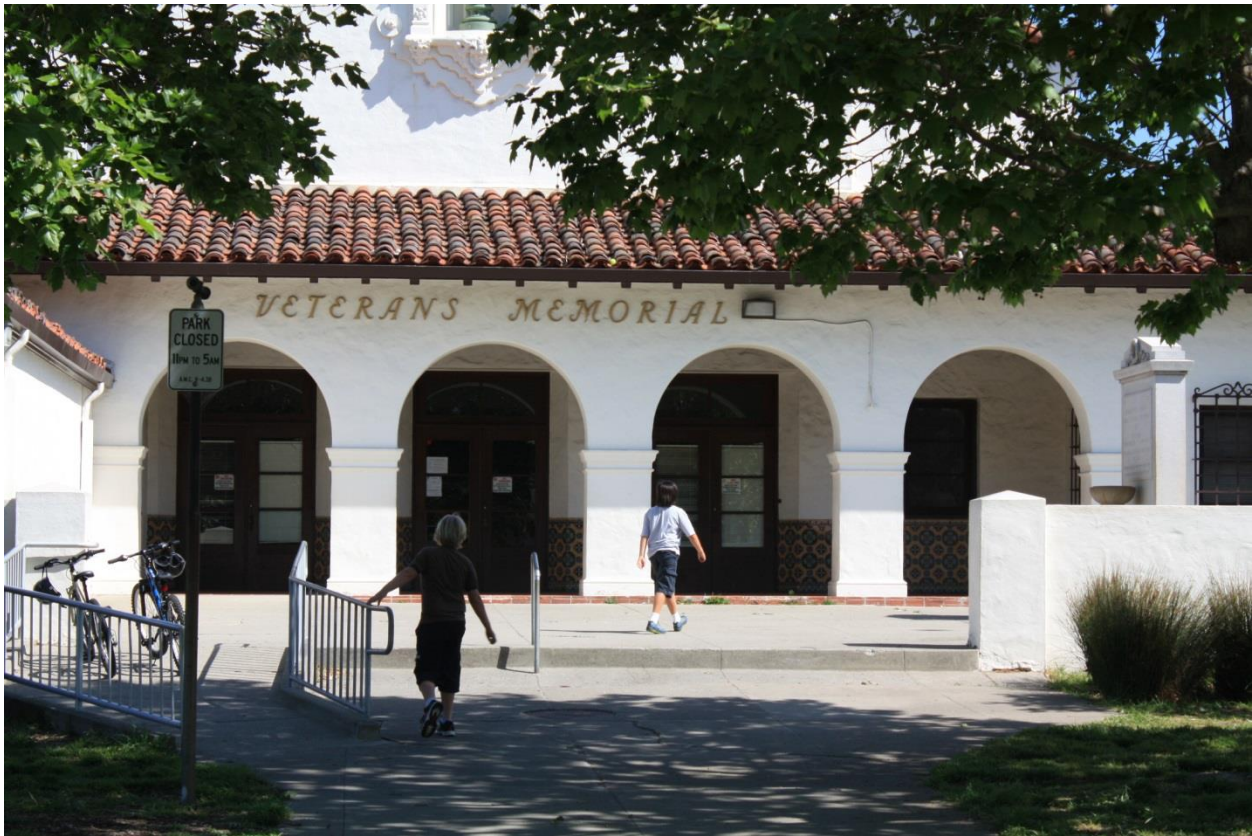
Veterans Memorial Building, Memorial Park
